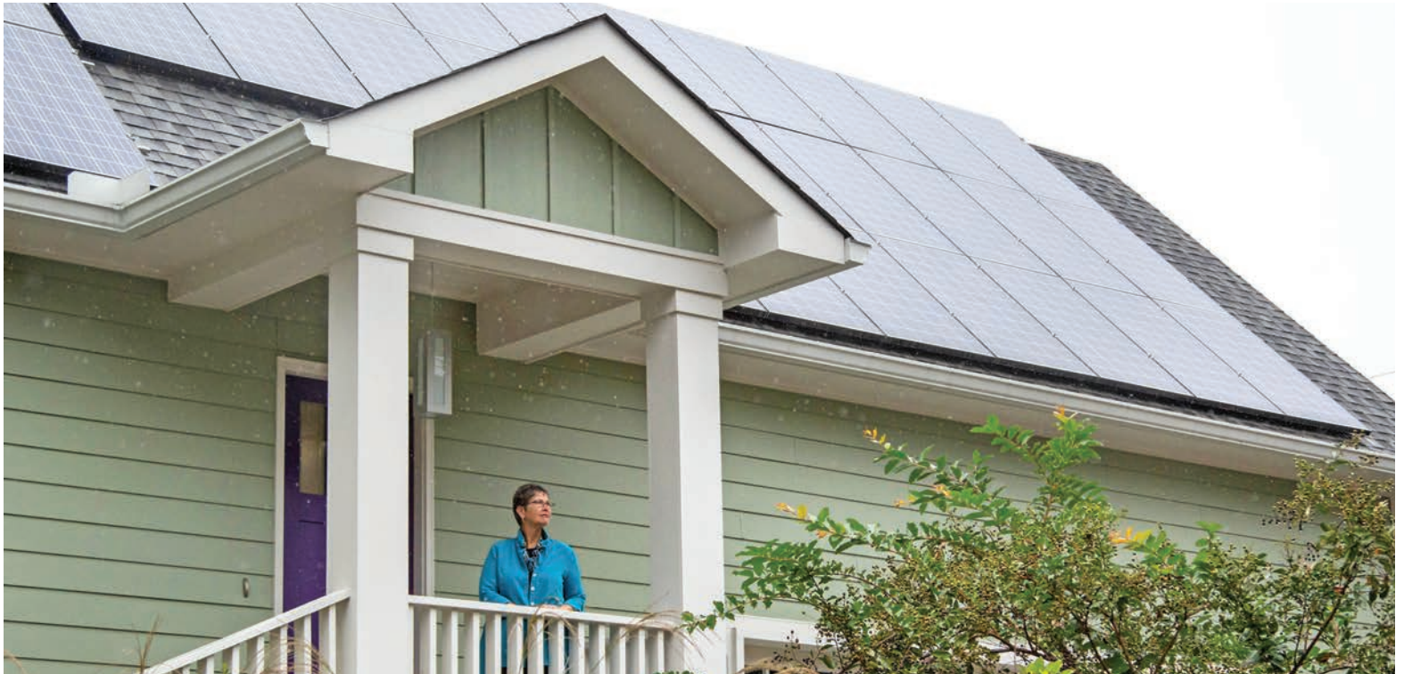
The largest LEED point generator for the Owens' green home was the installation of 42 solar panels.
